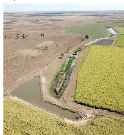
Aerial view of the water recycle pit
