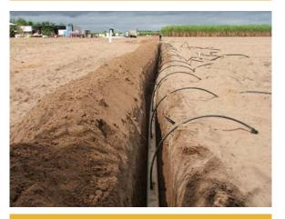
Underground pipes connect all the rows of irrigation equipment together
