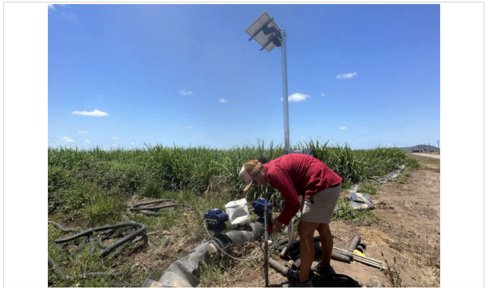
Installing irrigation control equipment
